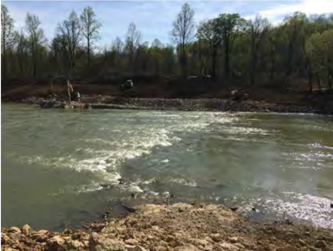
Green River, KY L&D 6 – Post Removal, 2017
