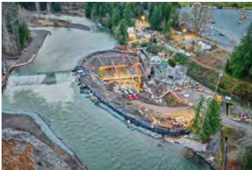
Mud Mountain Dam Fish Passage - $35M
